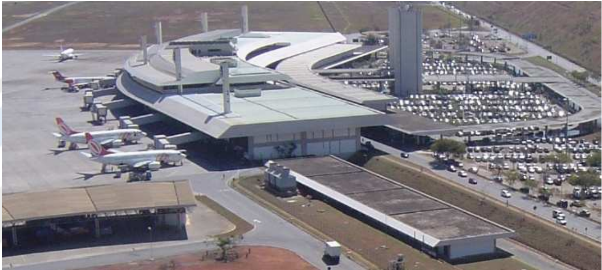
Figure 6 - Partial View of the Tancredo Neves International Airport
